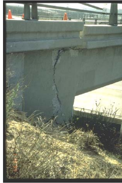
I-5/I-210, South交流道橋
